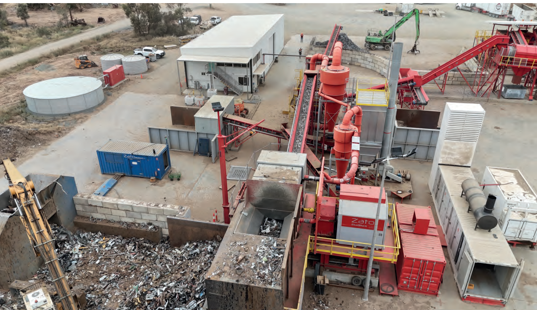
Access Recycling's main facility at Barmedman.
